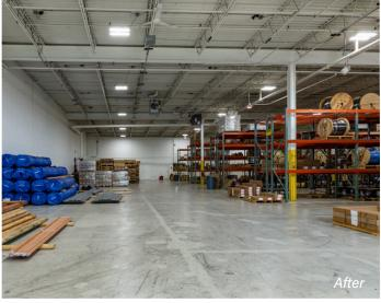
The warehouse replaced 178 six-lamp T8 fluorescent high bay fixtures with fewer than 60 Keystone 155W LED high bays, saving energy and providing more efficient lighting.
