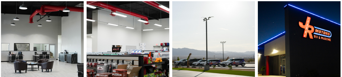
JR Motors used a variety of different Keystone products, pairing round high bays and wraps with exposed ductwork in the interior and using area lights for the parking lot and the Mistik DMX Wall Washer on the exterior.
